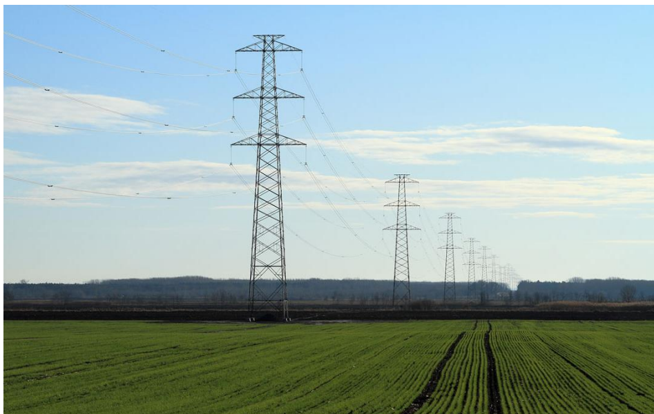
Figure 7.3.2-3: The Martonvásár-Győr 400 kV overhead transmission line with PINE towers
