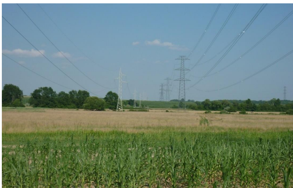
Figure 7.3.2-4: The Pécs-National Border 400 kV overhead transmission line with PINE towers, line corridor
