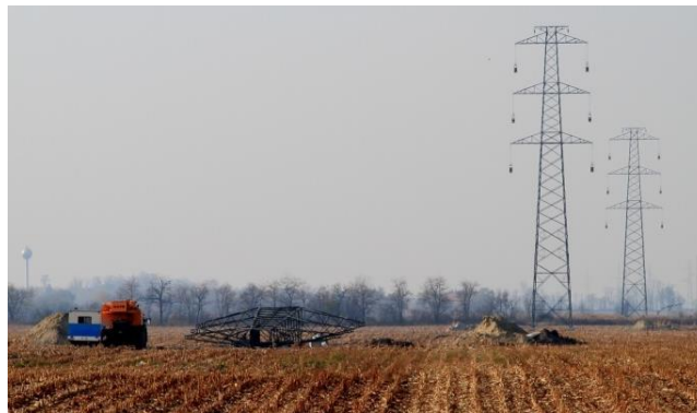
Figure 7.3.5-1: Martonvásár-Győr 400 kV overhead transmission line, space required for the assembly and erection of towers
